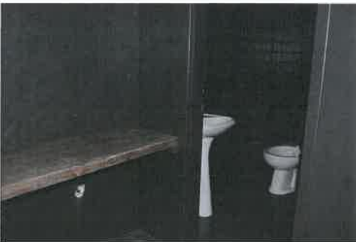
Sub. 3 Piano terra bagni
